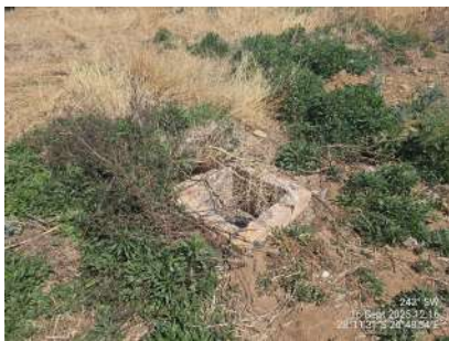
Conservancy tank to be removed.
