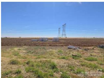
Materials to be removed from site camp.
