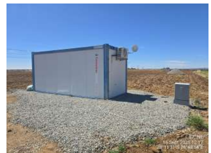
Container and aggregates to be removed.
