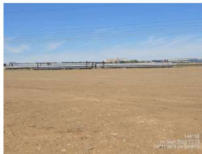
Equipment in laydown to be relocated.
