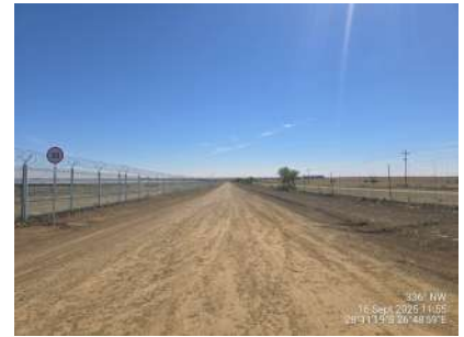
Perimeter road leading to O&M.
