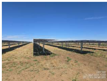
Panels installed on site.
