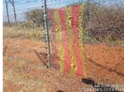
Fence where break in was reported is temporarily repaired.
