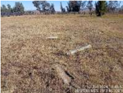
Building rubble on site.
