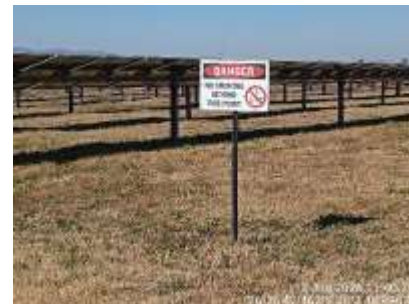
Safety signage, no smoking sign.
