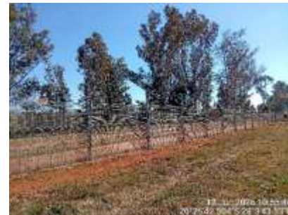
Fence and fire break adequately maintained.
