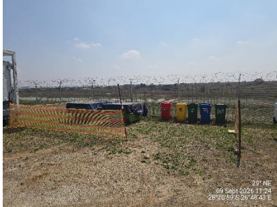
Waste bins at O&M building.
