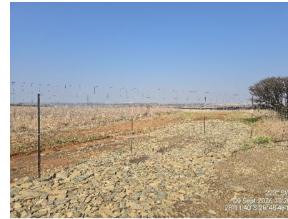
Vegetation clearance inside heritage site buffer area for stormwater control.
