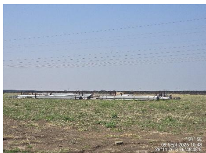
Equipment in laydown area to be removed.
