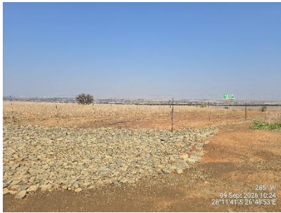
Vegetation clearance inside heritage site buffer area for stormwater control.
