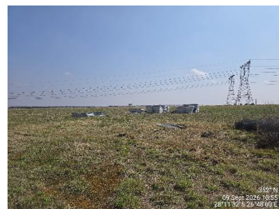
Equipment in construction site camp area to be removed.
