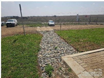
Grass planted and stormwater gabions at O&M.
