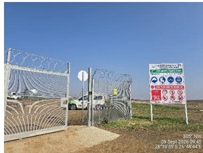
Access control into facility.
